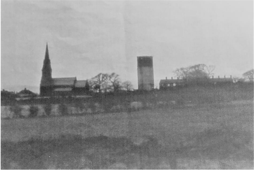
Figure 3: WUDC Water Tower (by permission of Alan Ravenscroft).
