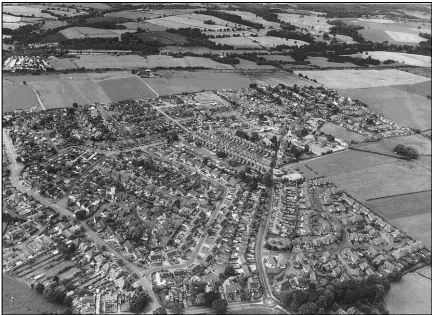
AERIAL VIEW OF MOULTON c.2000
