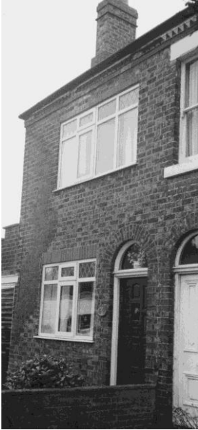
69, MAIN ROAD, MOULTON TODAY (2005)
